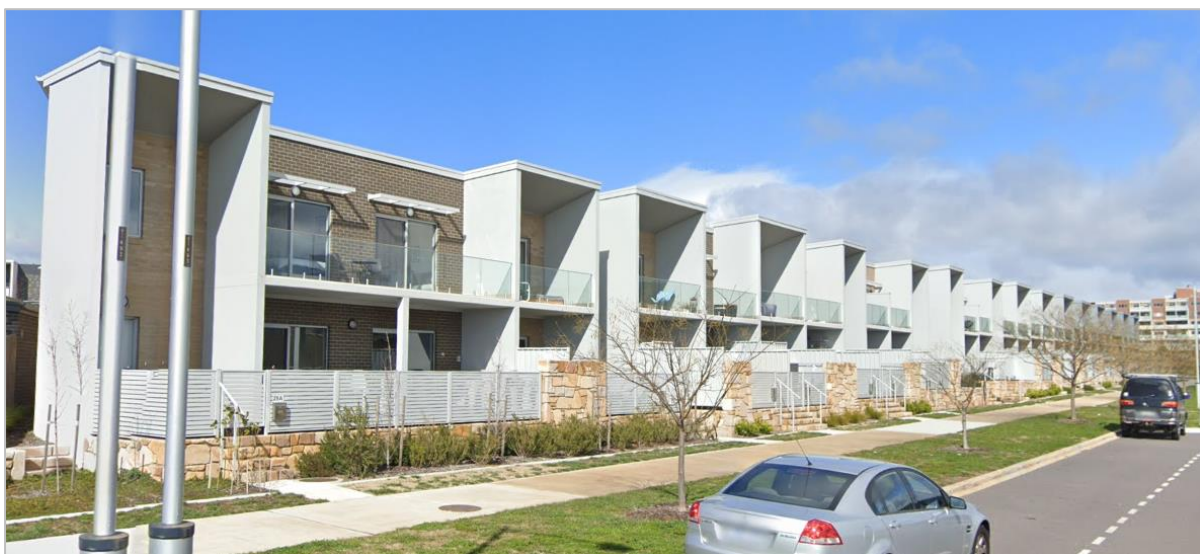
Figure 3: Residential developments at Coombs Section 7, Block 1 (top) and Section 41, Block 3 (bottom). Both sites are zoned “CZ5 Mixed Use”, but neither feature a genuine mix of uses.
